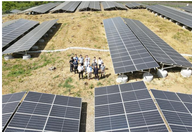
<Exterior View of the Power Plant in Kumagaya City, Saitama Pref.>
