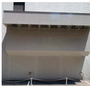
Raising of generator supply and exhaust ducts
