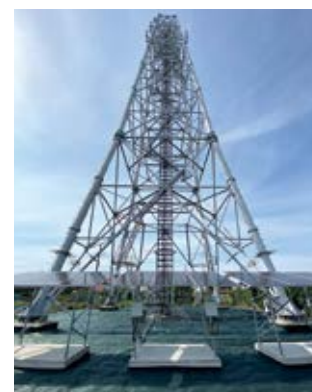
Solar panels installed at base stations
