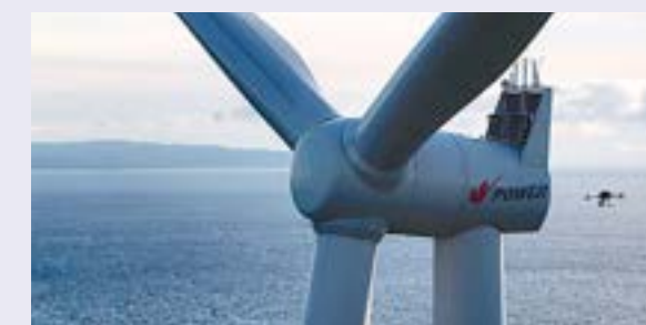
Autonomous flight drone efficiently performs inspections of offshore wind facilities.
