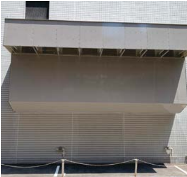
Raising of generator supply and exhaust ducts
