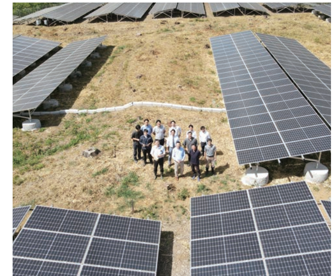
▲au Renewable Energy's first solar power plant
